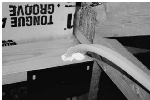
Sealed holes in a top plate as part of the airtight drywall approach.
