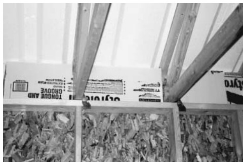
Raised-heel trusses bearing on an exterior wall top plate.
