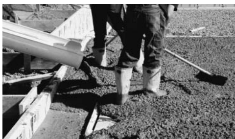
Constructing a frost-protected shallow foundation (monolithic slab as an integral footer, foundation, and floor).
